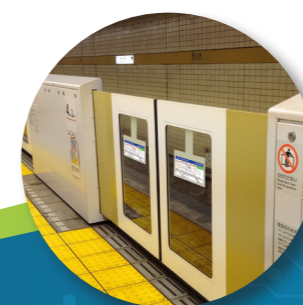
..... Passenger Screen Doors (PSD) .....
